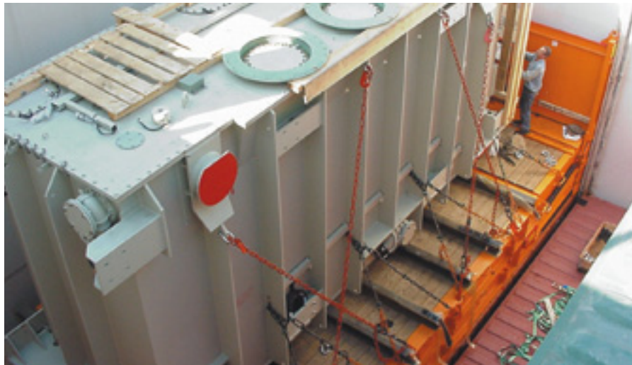
This transformer, weighing approx. 160t, was placed on steel girders and lashed with chains
