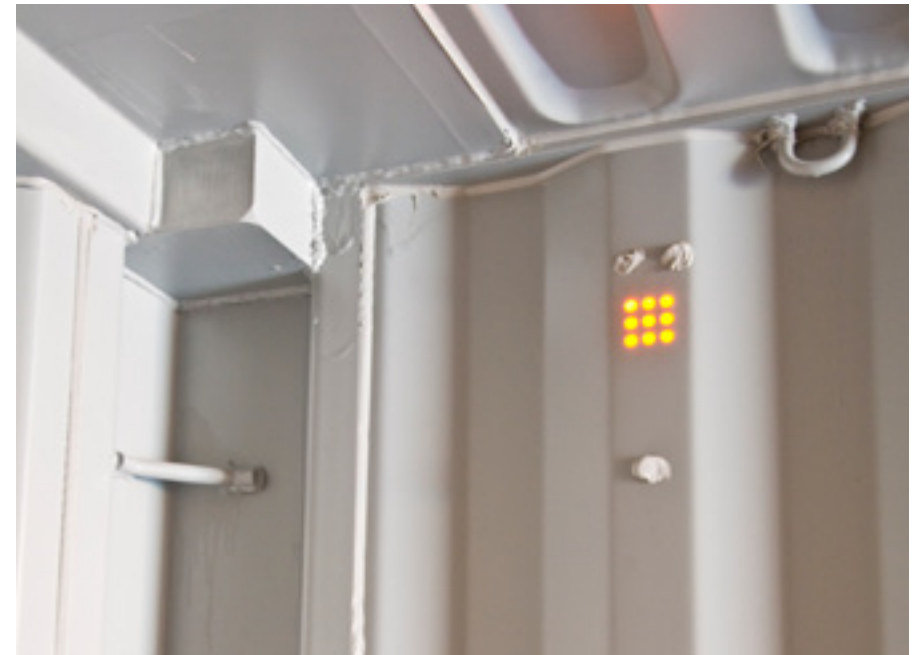
Lashing points in a standard container on the roof edge, at the corner post and small vents for air-pressure equalisation
